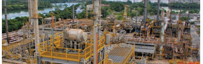
Ecopetrol Barrancabermeja Refinery Blue Hydrogen & Carbon Capture Colombia
